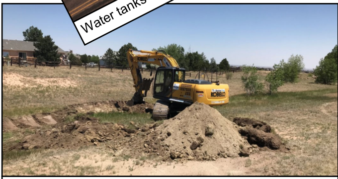
Filings 4 & 5 stormwater channel remediation.
