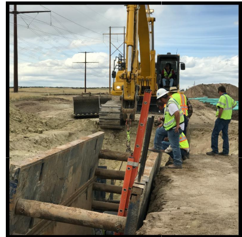
Excavation and installation of a sanitary sewer main.
