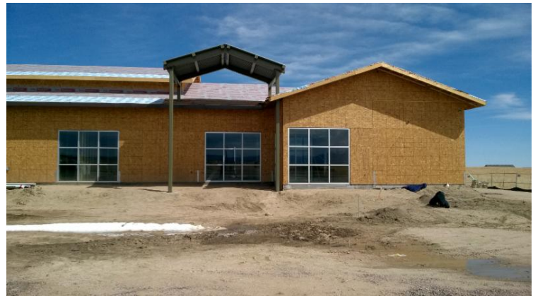
View of front entryway from Towner Ave.
