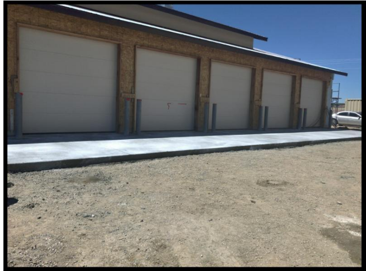
Maintenance area entry.
